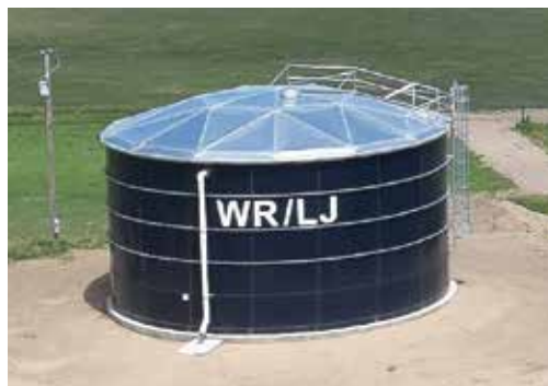
Newly constructed 300,000-gallon ground storage reservoir at Vivian.
