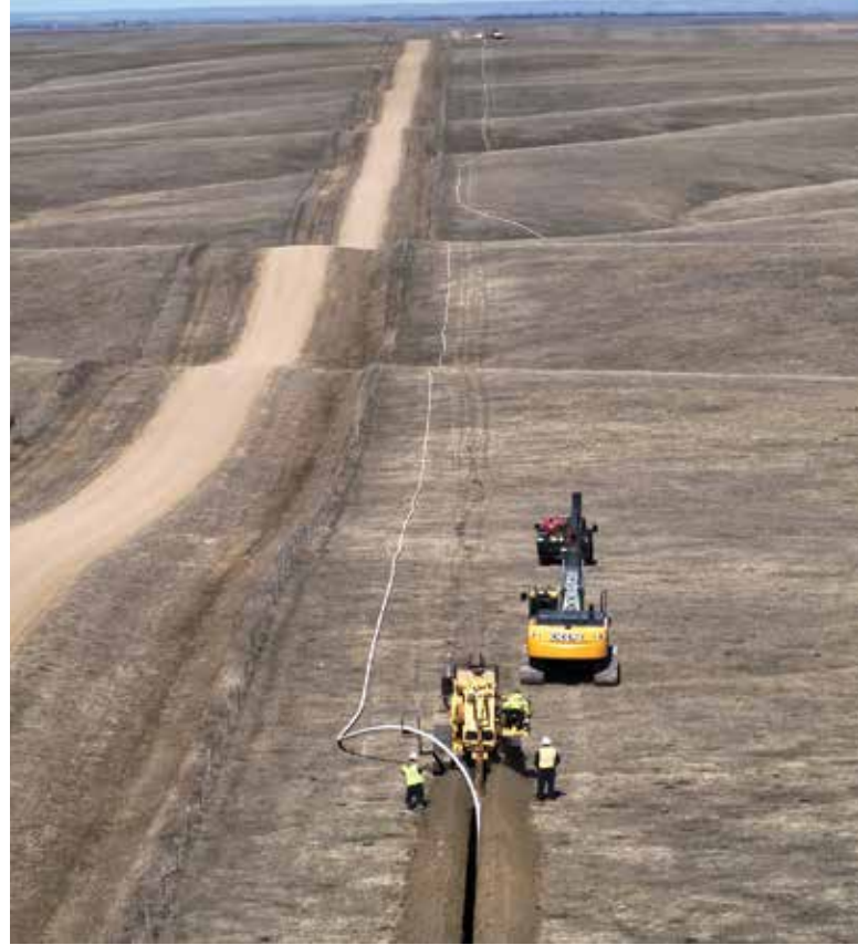
Pipeline installation in Haakon County.
