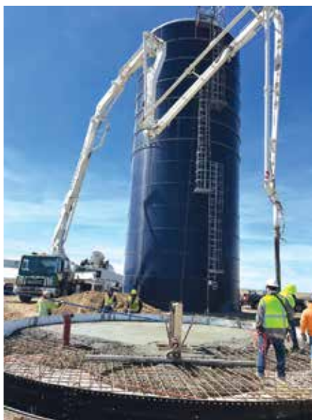
Floor slab being poured for the Creighton GSR.
